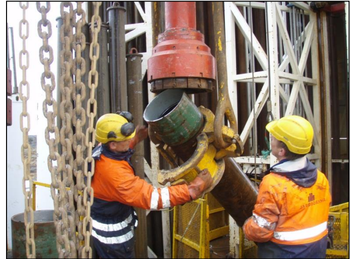
Casing brought up to drill-floor
